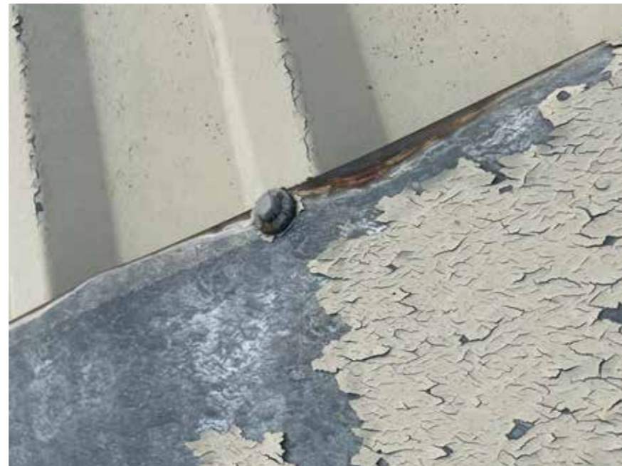
Carr Junior School roof before refurbishment
