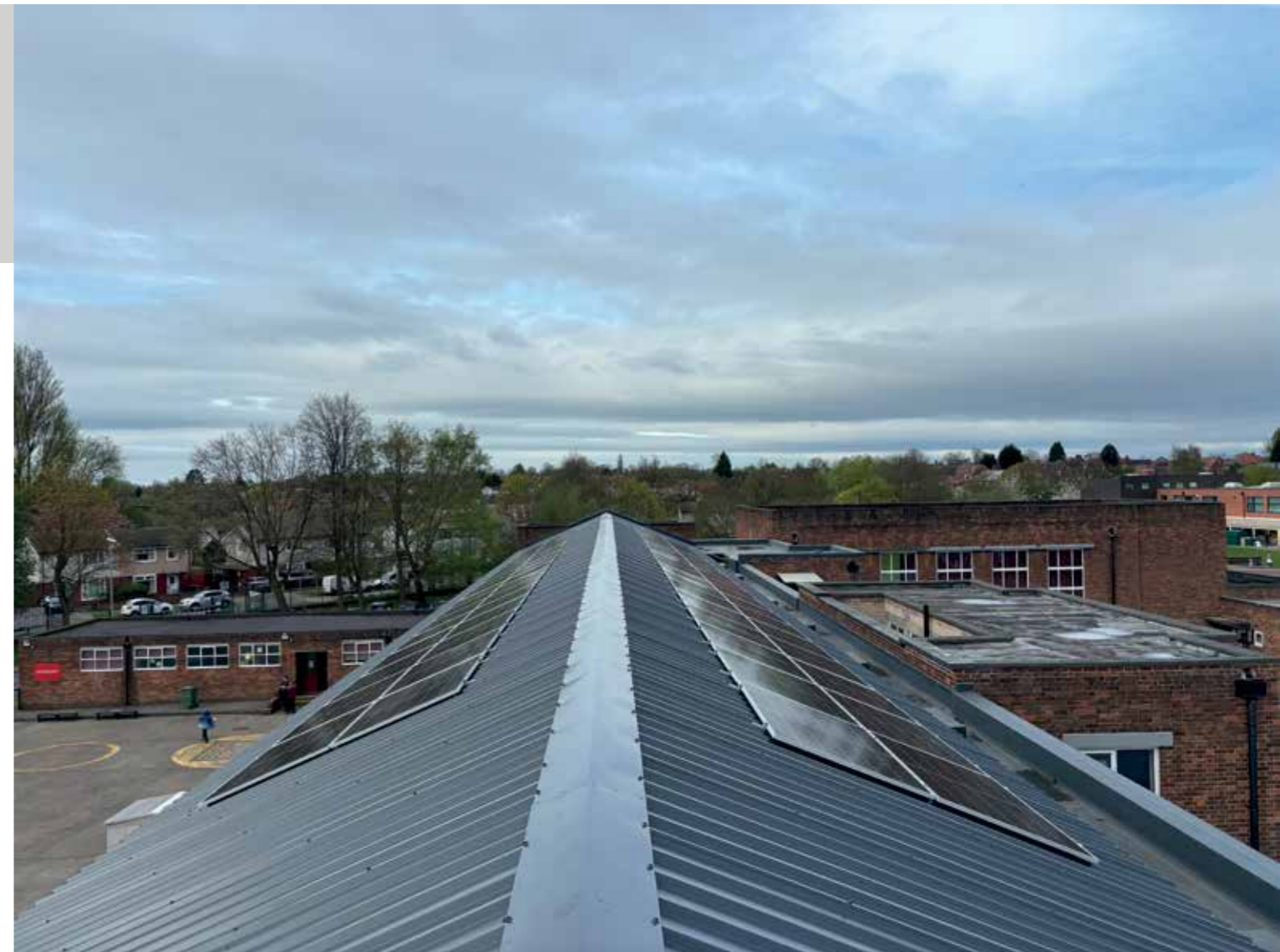
Carr Junior School roof refurbishment and Solar PV
