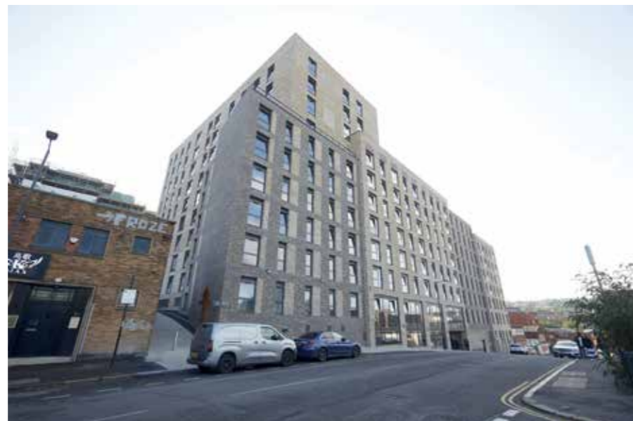
A newly developed residential complex utilising Heat Interface Units
